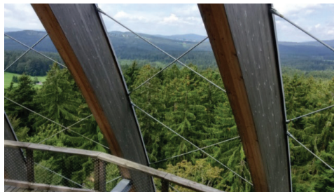
Figure 22-23. View from the inside of Treetop Walkway and the Glulam columns (URL-12)
