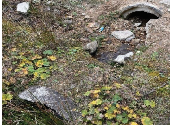
Figure 2. Example of structural failure in a culvert pipe caused by inadequate dimensioning
