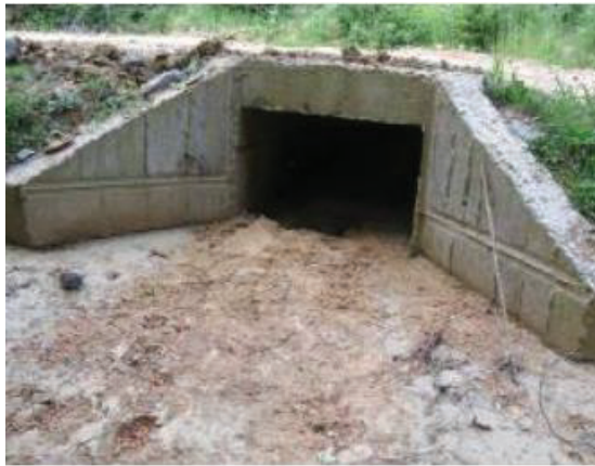
Figure 3. Example of a properly designed culvert in a forest road (Ozturk & Inan, 2010)
