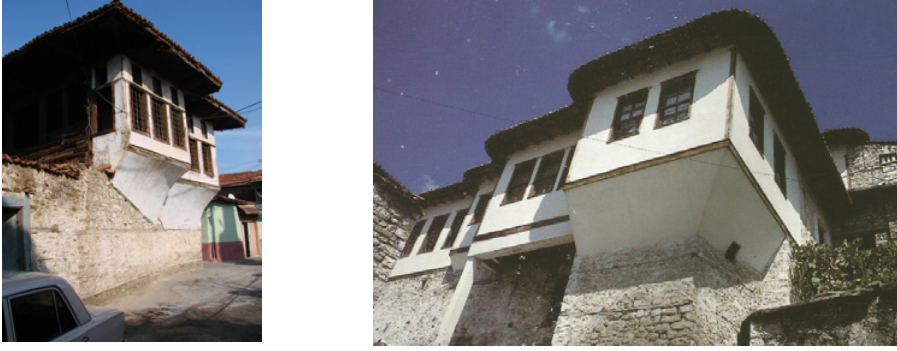
Figure 9 - 10. Composite construction system (downstairs is masonry and upstairs is timber frame), first Aegean Region in Anatolia, Manisa - Kula; second Berat - Albania.
