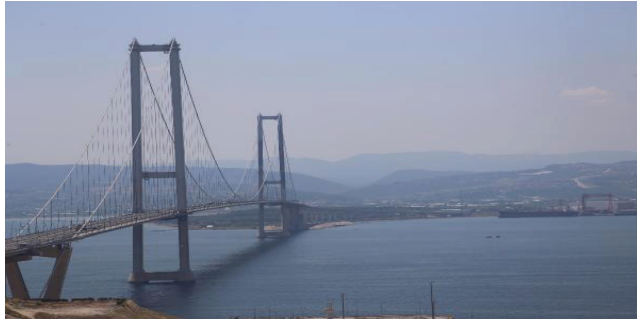
Figure 10. Osman Gazi Bridge
