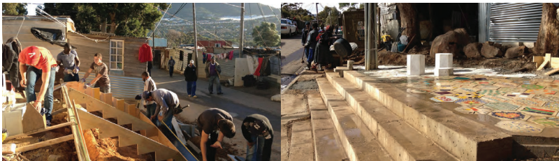
Figure 8. Platforms Construction (Louw, 2013)
