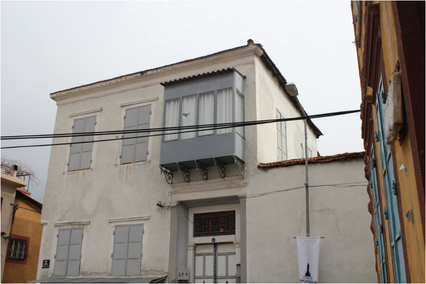
Figure 8: Current physical condition of the historical buildings.
