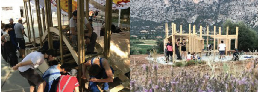
Figure 15. Fethiye, Kayadibi Village Playgrounds Construction Phase and Completed (Url-1).
