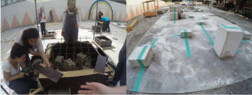
Figure 13. Ayazağa Primary School Playgrounds Construction Phase and Finished (Url-1).
