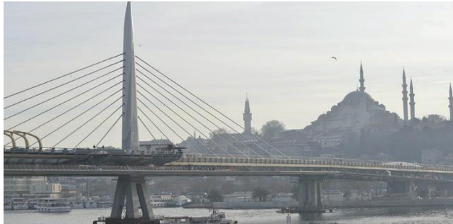
Figure 9. The Relationship between the historical peninsula and Golden Horn Metro Bridge
