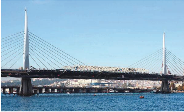
Figure 8. The Golden Horn Metro Bridge
