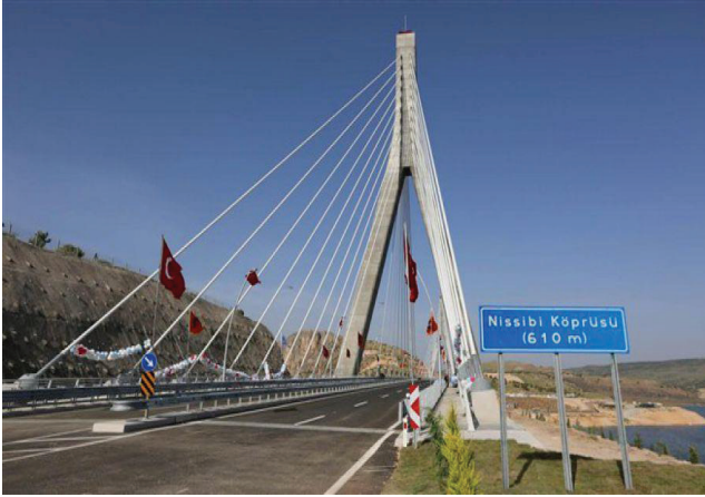
Figure 7. The Surface Texture of Nissibi Bridge
