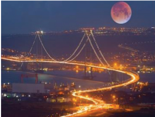
Figure 11. The lighting of Osman Gazi Bridge
