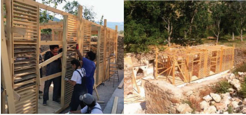
Figure 16. Merzifon Rest Station Construction Phase and Finished (Url-1).
