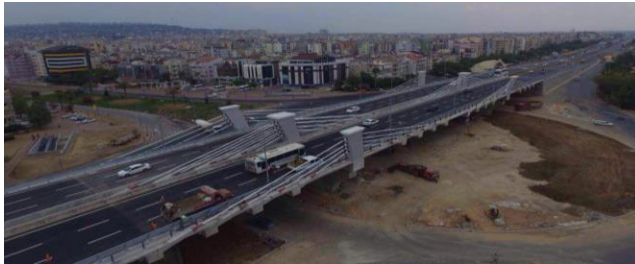
Figure 4. The Calli Bridge
