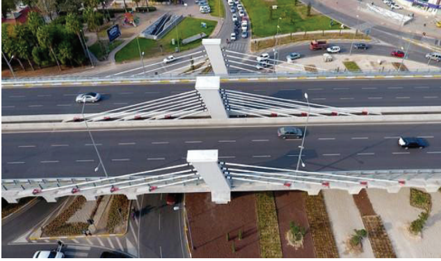
Figure 5. The Integration of Çalli Bridge into Environment
