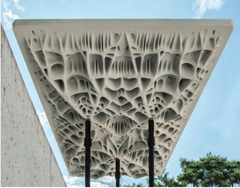
Figure 10 3D-Printed Stay-in-Place Formwork by ETH Zurich (Jipa et al., 2016)
