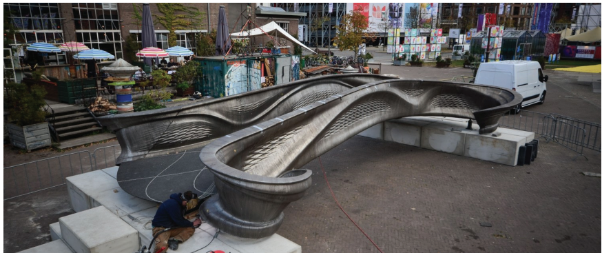
Figure 13 3D Printed Bridge by MX3D (Gardner et al., 2020)
