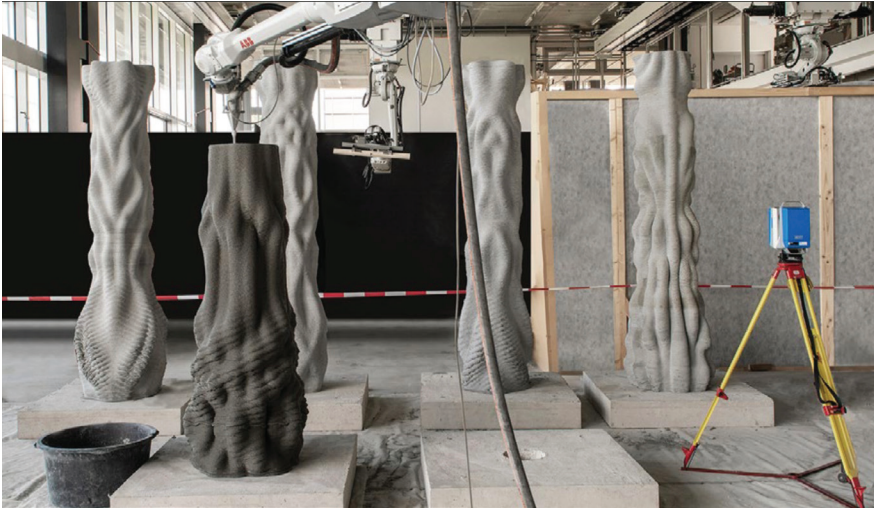
Figure 12 Concrete Choreography by ETH Zurich (Anton et al., 2020)
