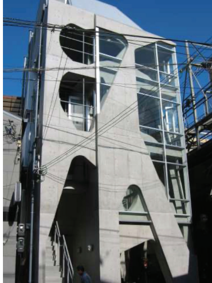
Figure 5 Akutagawa River Side Office Building in Takatsuki, Japan, 2004 (Omori & Ohmori, 2008)
