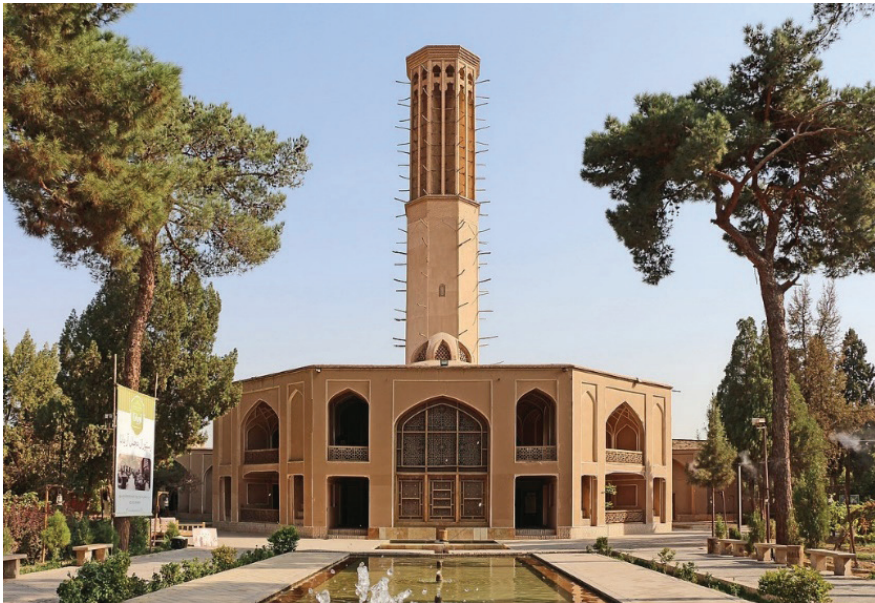
Figure 3.12: Wind tower in Dolat-Abad Garden, Yezd, Iran (Url-6).
