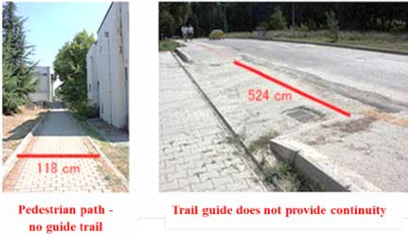
Figure 4. Pedestrian roads and sidewalk - guide track relationship in the example of education faculty and dormitories region (Hanik, 2019 – Original)
