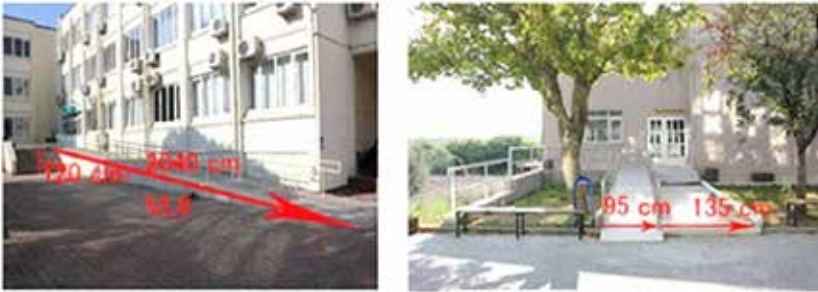
Figure 7. The ramp-stair relationship in the example of the Faculty of Arts and Sciences (Hanik, 2019 – Original)
