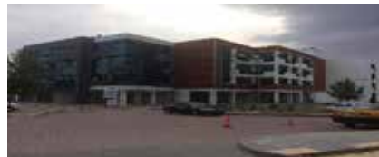
Figure 17. Image from the Finished Building
