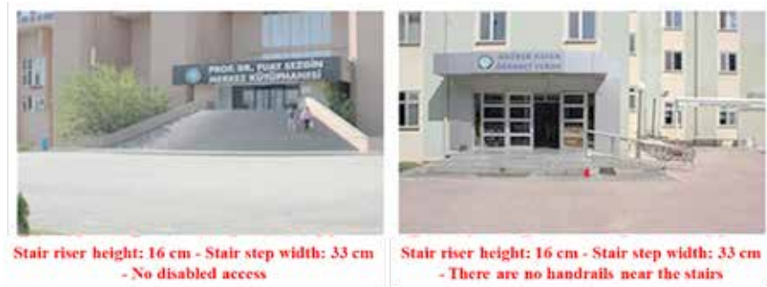
Figure 9. Bursa Uludağ University, in front of the central library and dormitories area building-stairs relationship (HANİK, 2019 - Original)
