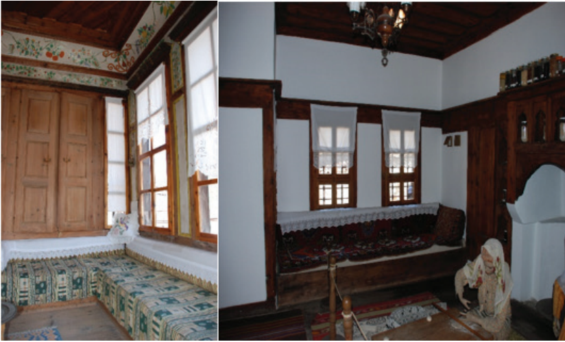
Figure 11. Reinforcement Elements Shaped Together with the Building in Traditional Turkish Houses: Cedar, Wardrobe and Niches (Demirarslan, 2011).
