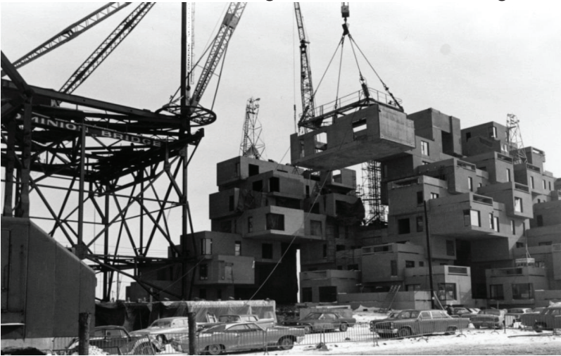
Figure 6. The on-site construction stages of concrete modular blocks by using lifting vehicles ( https://www.arkitektuel.com/habitat-67/ ).
