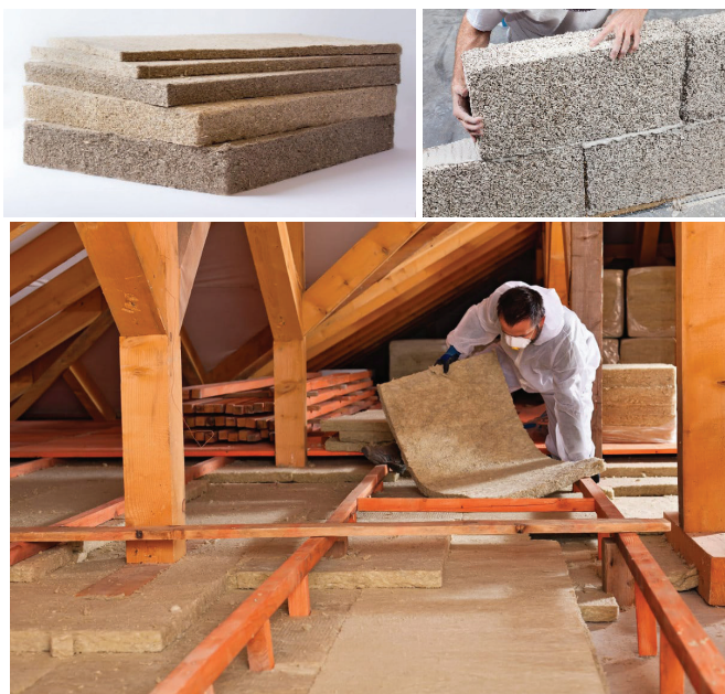
Figure 14. Thermal insulation applications with hemp fiber [33-35]
