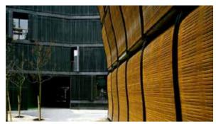
• The use of materials that absorb sound or reduce sound pressure on the façade reduces sound transmission.
