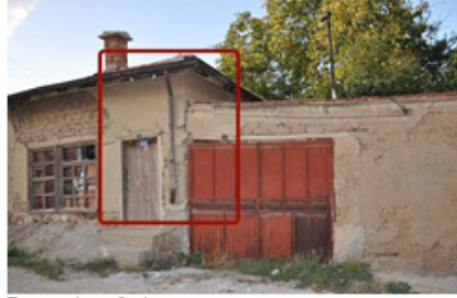
Renovation of rain gutters
