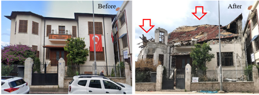
Fig. 17. Before earthquake (Google Street View, 2022) situation b. After the earthquake situation of the historic building of the Union of Chamber for Merchants and Craftsmen in Antakya, Hatay
