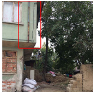
Renovation of rain gutters
