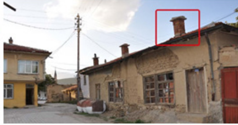
Renovation of chimneys
