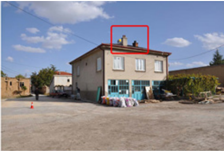
Repair and cleaning of chimneys
