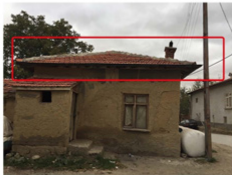
Repair of roofs with pantile type tiles
