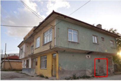
Repair of distortions on facades with plaster
