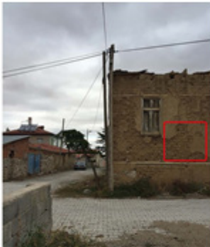
Repair of facades with adobe plaster
