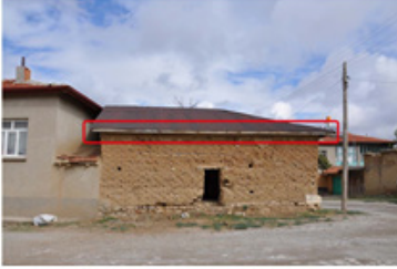
Renovation of roof pediments
