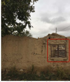
Renovation of railings with knotted iron grille
