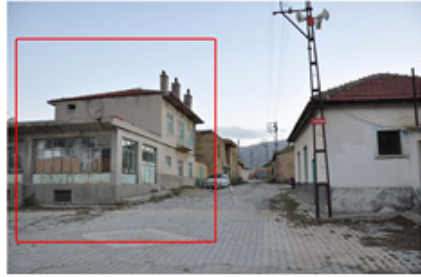
Completion of structures without a roof with marseille-type tiles
