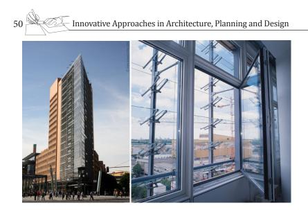
Figure 1. Berlin Debis Tower (Left-hand side) (URL-1)Figure 2. Double facade of the building with operable window inside, and an outer<br/>glazed skin (Right-hand side) (URL-2)
