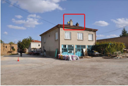
Repair and cleaning of chimneys
