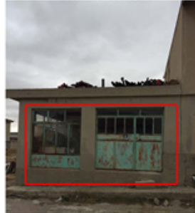
Renovation of door joinery with wooden-looking aluminum material
