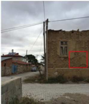
Repair of facades with adobe plaster
