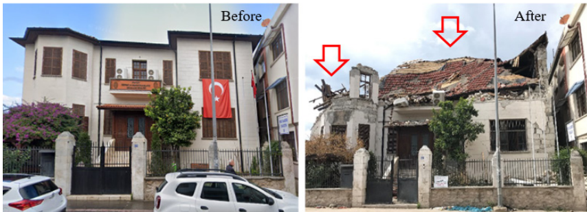
Fig. 17. a. Before earthquake (Google Street View, 2022) situation b. After the earthquake situation of the historic building of the Union of Chamber for Merchants and Craftsmen in Antakya, Hatay
