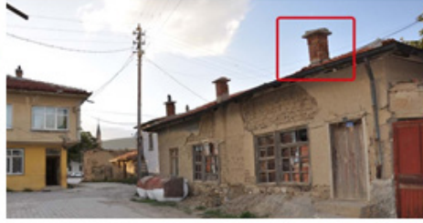
Renovation of chimneys
