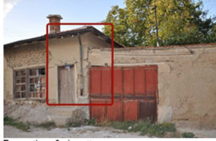
Renovation of rain gutters
