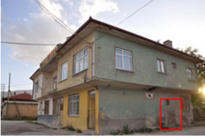
Repair of distortions on facades with plaster
