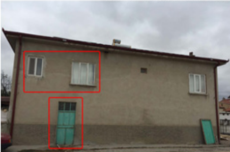
Renovation of window joinery with pvc material with wooden appearance
