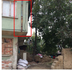
Renovation of rain gutters
