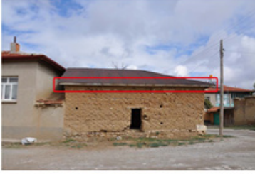
Renovation of roof pediments
