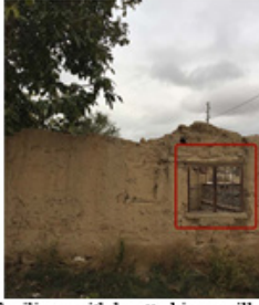
Renovation of railings with knotted iron grille
