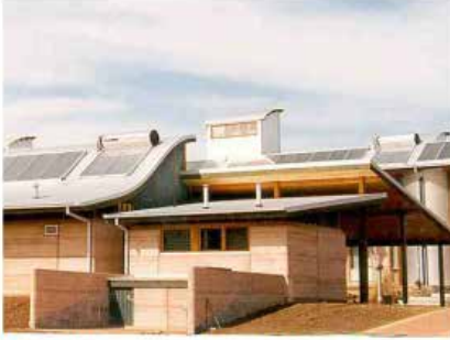
Illustration 3.71: Composting toilet basement (1999)
