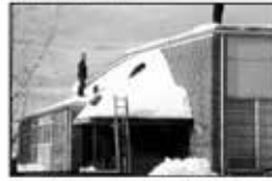
Figure 4. The peak snow load of this drift was 130 psf. The ground snow load at the time was 20 psf, and the snow load on the upper roof was 15 psf.
