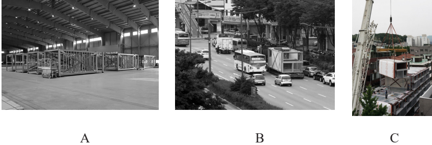
Figure 11. Construction phase of Hadaewon Residences
