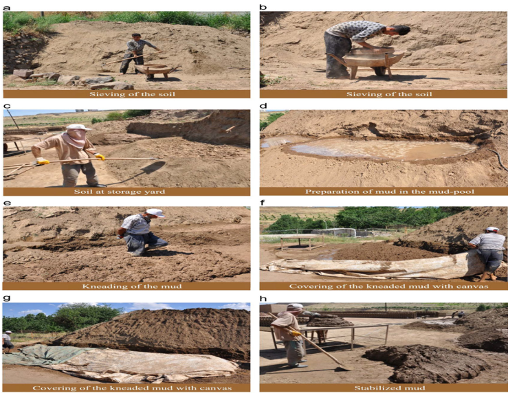
Figure 4. Production process of adobe mixture (29)
