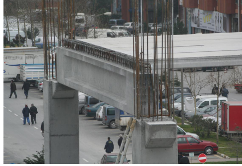
Figure 16. Prefabricated beams and hollow floor elements placed on cast-in-place columns (Özkan, 2003).
