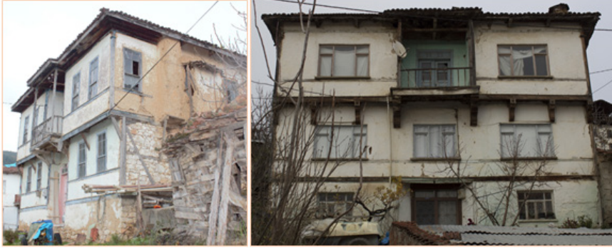
Figure 27. Examples of houses with balcony overhangs on the middle axis of the facade on the top floor on the front facade and room overhangs on both sides of the balcony
