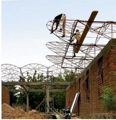
(Figure 8). Dano Secondary School Canopies (Url 1).
