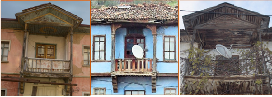
Figure 31. View of the roof eaves on the balcony, complete with flat or gable pediment
