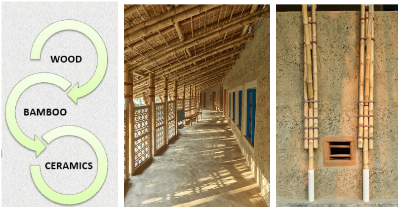
Figure 20. Rudrapur Community Center and Workshop Complex Materials (Url 6).
