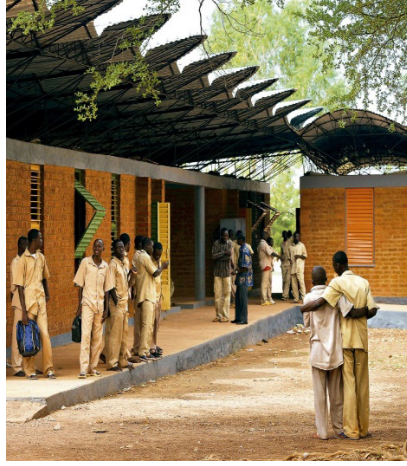
(Figure 10). Danu Secondary School Roof (Url 1).
