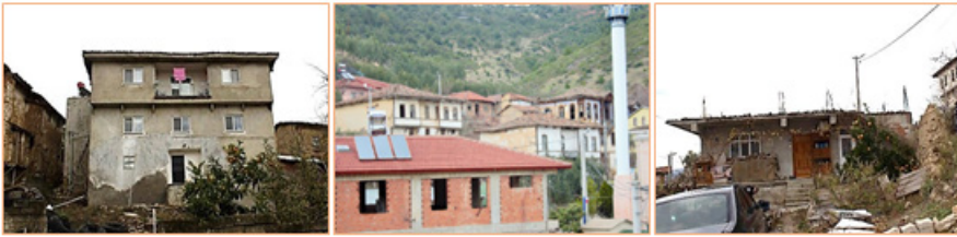
Figure 5. View of buildings built in reinforced concrete style within the texture
