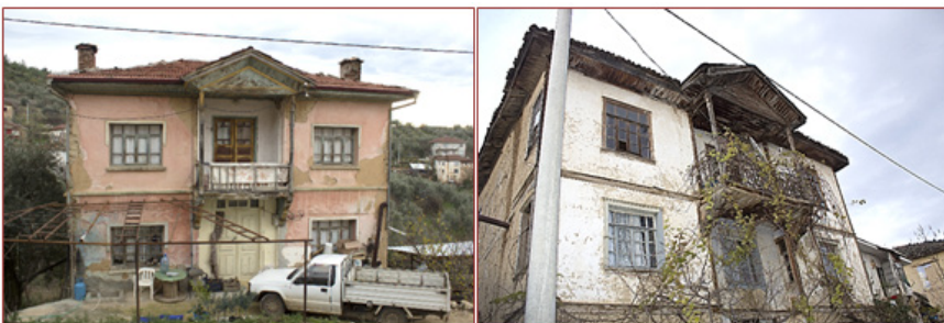
Figure 28. Examples of houses with only balcony projections on the front facade
