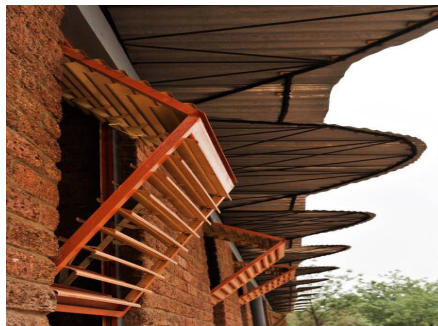
(Figure 12). Dano Secondary School Windows (Url 2).
