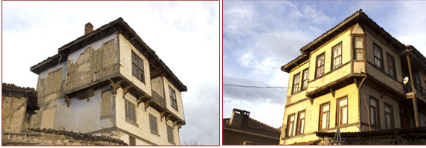
Figure 29. Examples of houses with protrusions on the street and side façades, joining each other at right angles or at a 45-degree angle
