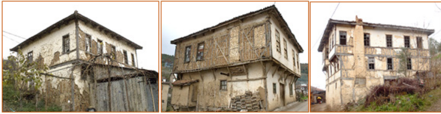
Figure 30. In the local texture, examples of houses from the Ottoman period where the front facade is completely projected, the front and side facades are projected, the middle axis of the front facade is not projected, and both sides are projected
