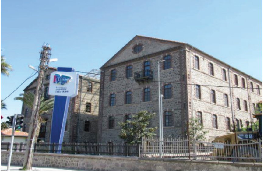
Figure 5. Halkapınar Flour Factory - Fabrication Lab (FabLab) (Ünal, 2020).
