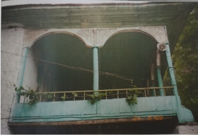
Photo 1. East facade of Kırkoluk Mosque, (Photograph taken by Başak KatranCI,2003)
