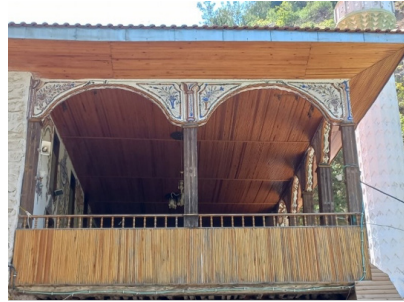
Photo 3. East facade of Kırkoluk Mosque, (Photograph taken by Başak KatranCI,2022)
