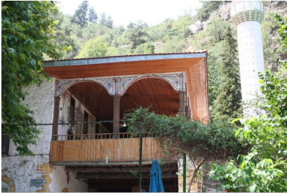
Photo 2. East facade of Kırkoluk Mosque, (Photograph taken by Başak KatranCI,2017)
