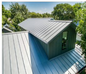
B. Metal roof
