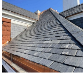
D. Slate roof
