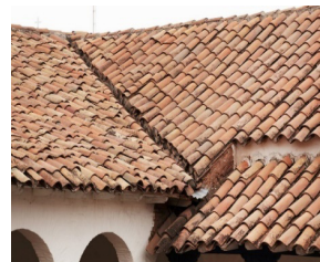
C. Clay tile roof
