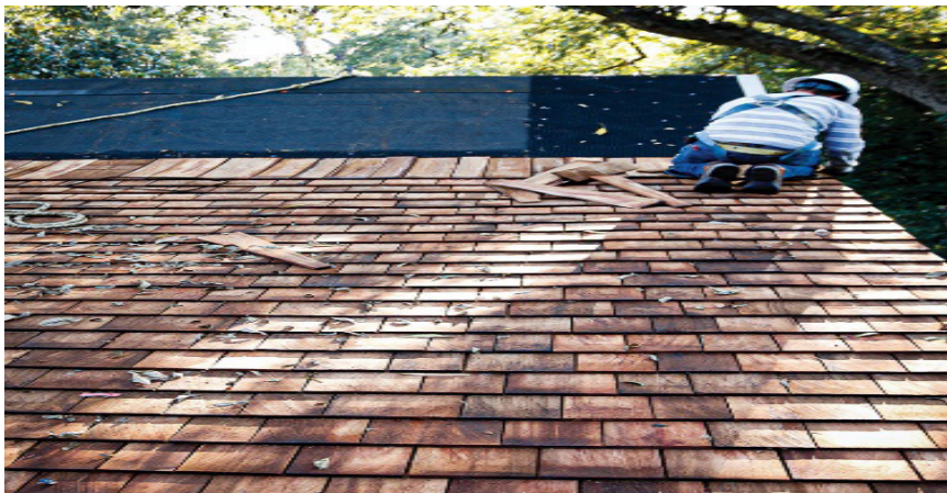
Figure 3. Wood shingle roof with cedar breathes
