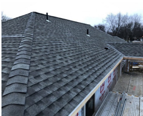
A. Asphalt shingle roof
