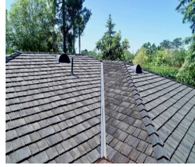
E. Concrete tiles roof
